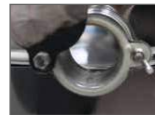
Gate AISI 304 Stainless Gate Welded on lowest level
